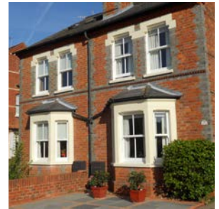
Wood stained timber framed top-hung casements (installed some 30years ago) were replaced with sliding box sash.
