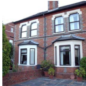
Wood stained timber framed top-hung casements (installed some 30years ago) were replaced with sliding box sash.
